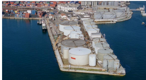
Fig.2 Petrolig Genova Plant
